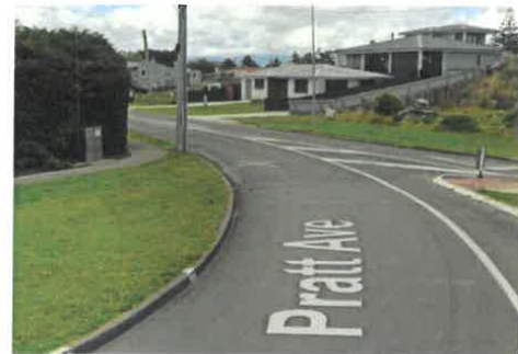
Figure 7: Pinch point at Carthew Tce roundabout
