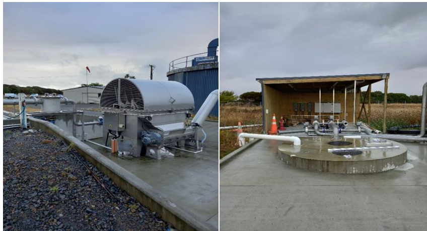
New septage receiving station
