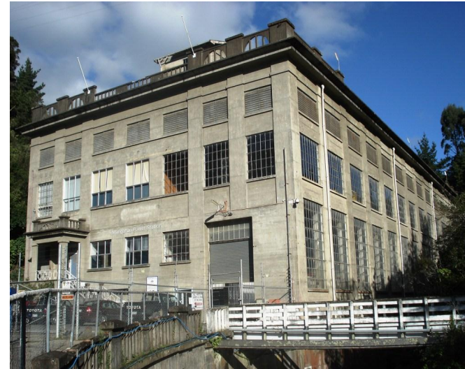
Figure 2: Mangahao Hydro-electric Power Station; courtesy of the Te Horowhenua Trust
