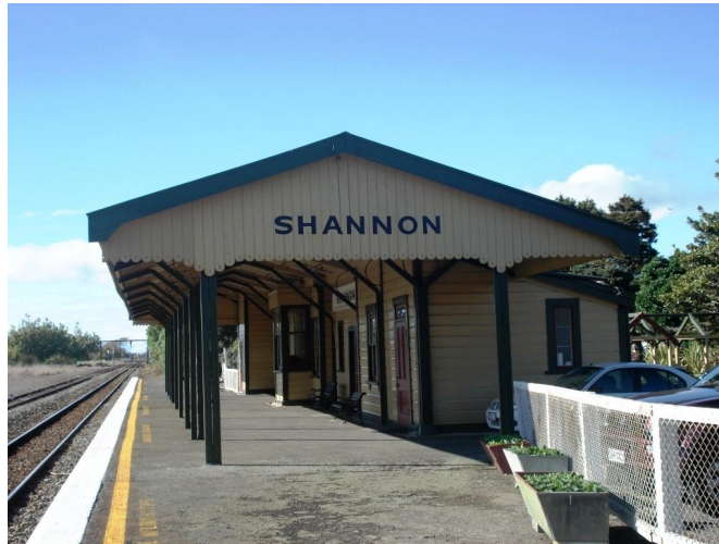
Figure 3: Shannon Railway Station; courtesy of the Te Horowhenua Trust
