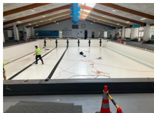
Installation of new pool liner
