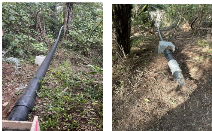
WW pipe renewal works Mangaore Village, Shannon
