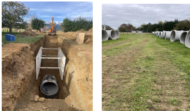
Stormwater pipe materials and installation at the Okarito site Levin.
