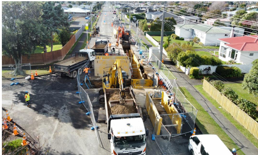
Sewer bulkmain works Tiro Tiro Road Levin
