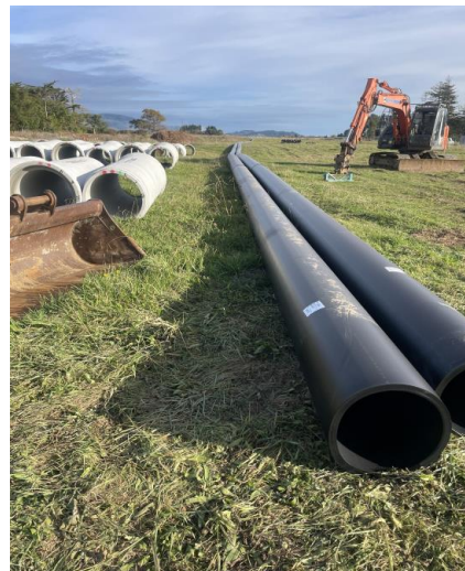
Queen Street WW pipe lengths after welding completed
