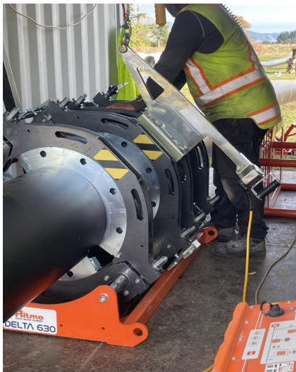
Queen Street WW pipe welding
